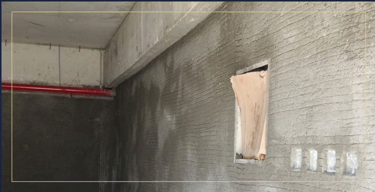
10 Plaster and electrical rough-in
