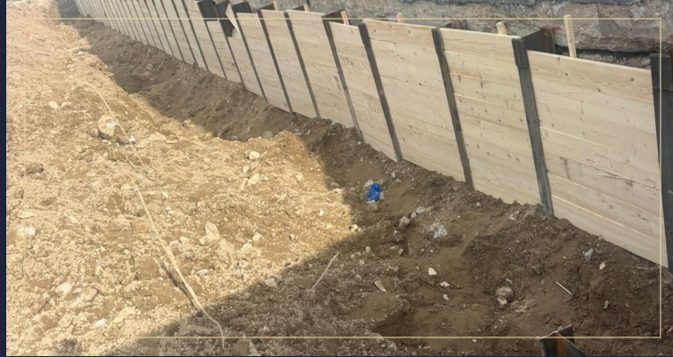
2 Excavation and shoring
