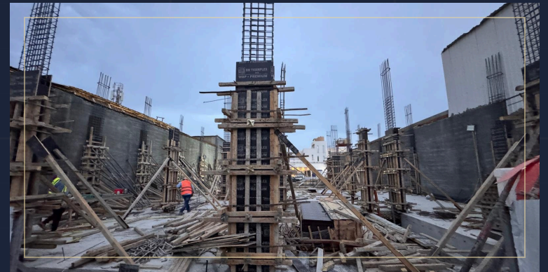
6 Column formwork
