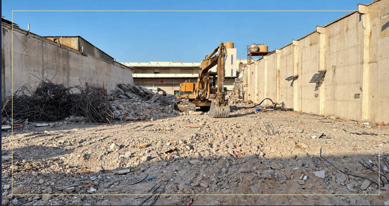
1 Demolition and site preparation
