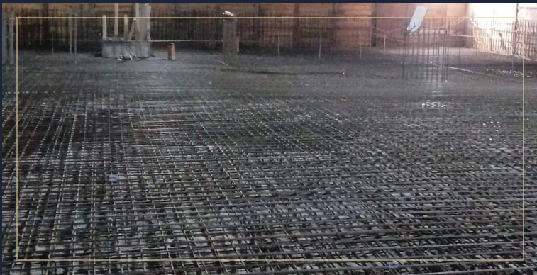
4 Foundation reinforcement
